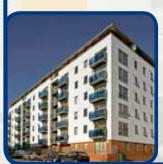
NCC recommended and supplied a fast setting solution with a SBR polymer modified screed, which was laid to falls, followed by a broadcast resin bonded deck surfacing system from Ronacrete, which was similar to the one used on the Tyne Ped. This was finished with decorative, light grey and slip resistant aggregate. All the 34 individual balconies, totalling an area of 269m<sup>2</sup>, were completed on time and to budget.
